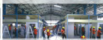
INTERIOR DRY WALL INSTALLATION
